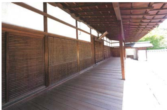
plate 2 structures and shadows of the eaves, Tofuku-ji temple (Naoki OUE)
